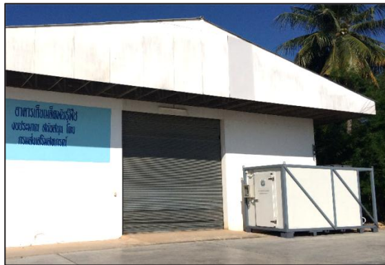
Figure 16 Container testing at Ni KhomLansak Cooperatives
