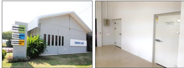
Figure 7 Cold storage room (Seed lab)
