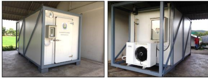
Figure 6 Cold storage room (Container)
